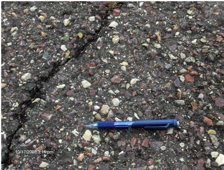
Raveling and weathering are the wearing away of the pavement surface. Raveling is the condition where the mid- to large size aggregates are becoming dislodged; weathering is when the fine aggregate wears away exposing the edges of the larger aggregate. These distresses are usually evident over large areas and may occur together (pictured above) or separately. Raveling and weathering may indicate that the asphalt binder has hardened significantly.
